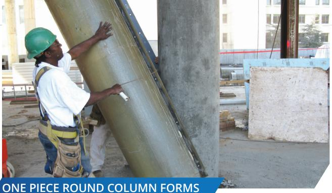
Round column forms, as they are typically referred to, are made from fiberglass making them dent, sag and rot resistant with minimal maintenance. Round column forms for rent or sale come in standard sizes 12" to 48" diameter. Additional sizes are quoted upon request.
