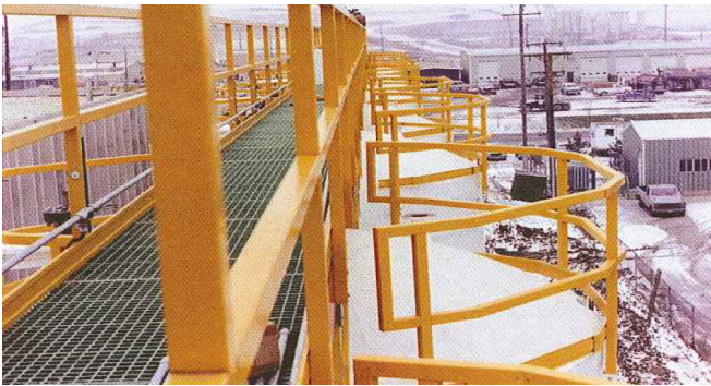
Internal connections make circular handrail systems such as these possible around tanks.
