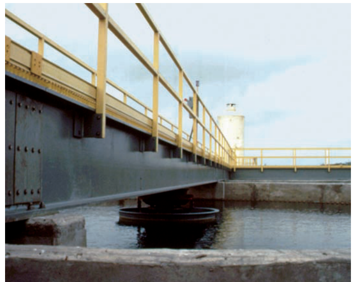
Lightweight, corrosion resistant 24" (610mm) I- beams span 45' (13.7m) to bridge clarifiers at the Las Rusias, Texas Wastewater Treatment Plant.
