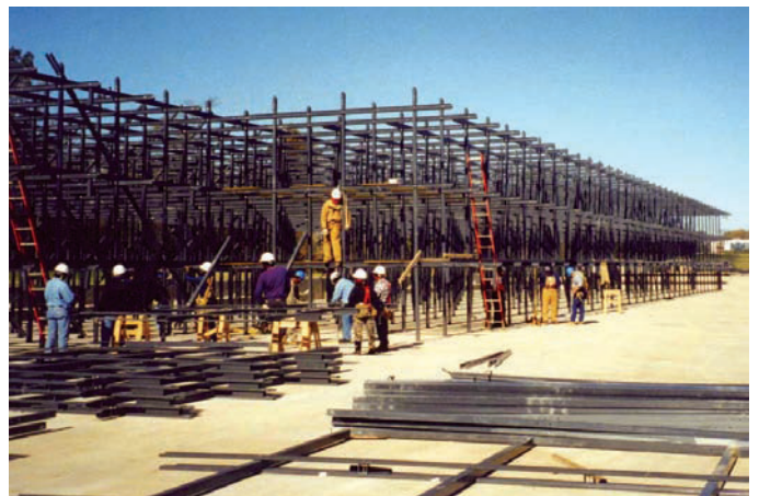
EXTREN® does not rot or corrode; making it the ideal material for cooling tower construction.
